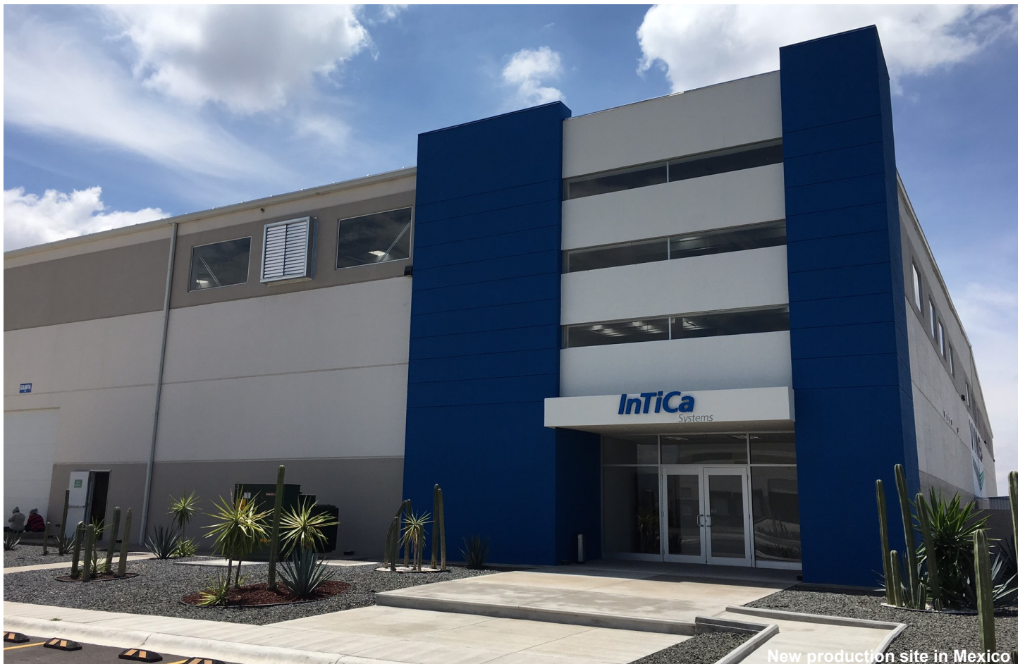
New production site in Mexico
